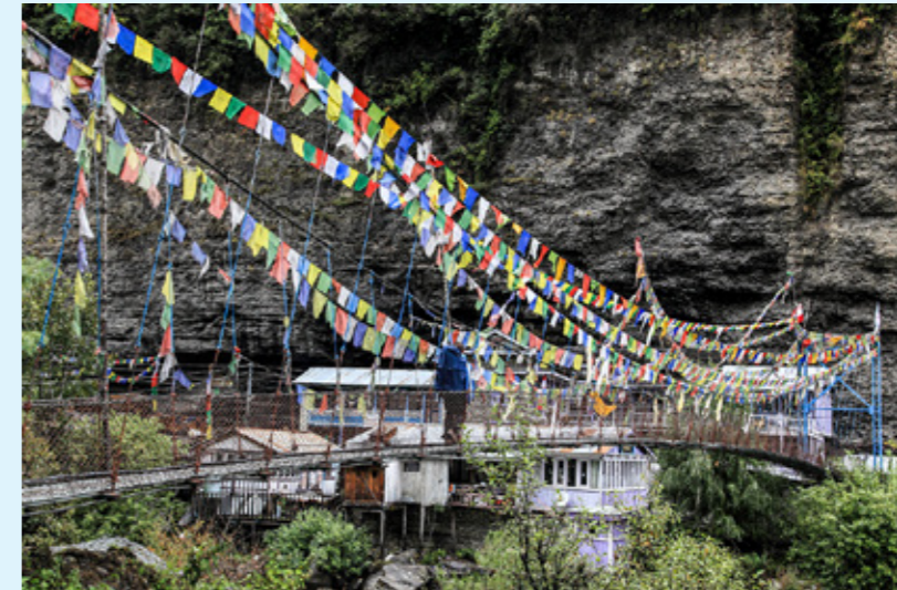
Hanging bridge, Pisang
